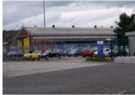
Longsight railway shed, SJ869960, 17.6.2019
