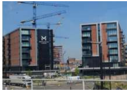
Former Hampson Street trading estate, 16.5.2019
