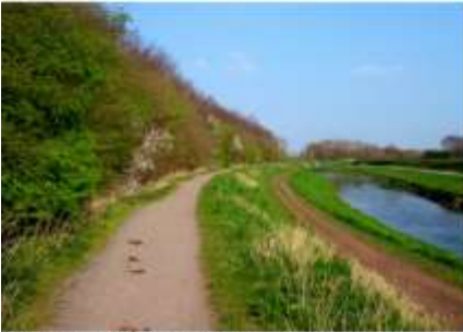
W. of Stretford sewage farm, SJ7793, 1.4.2007: flood-defence banks provide S-facing grass habitat
